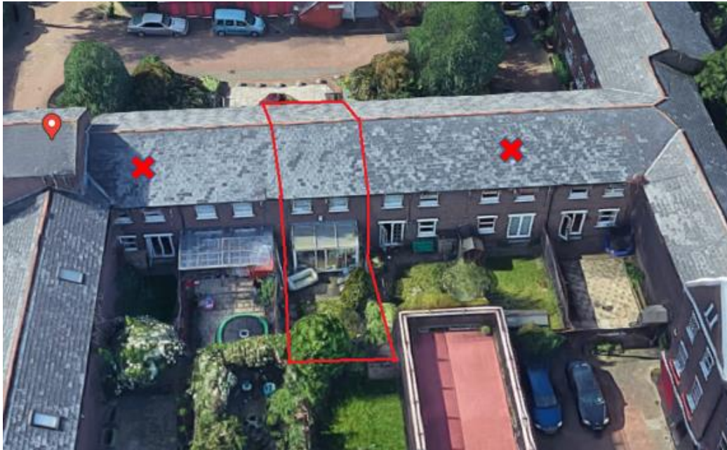
Figure 4: Rear elevation of the terrace
