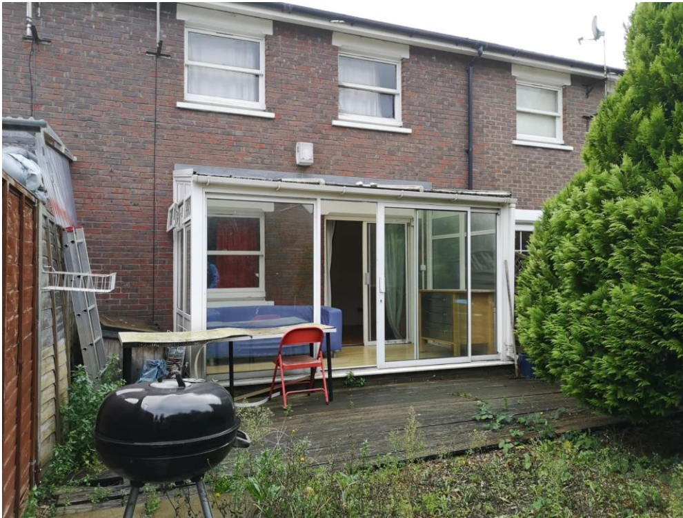
Figure 2: Rear elevation of the application site
