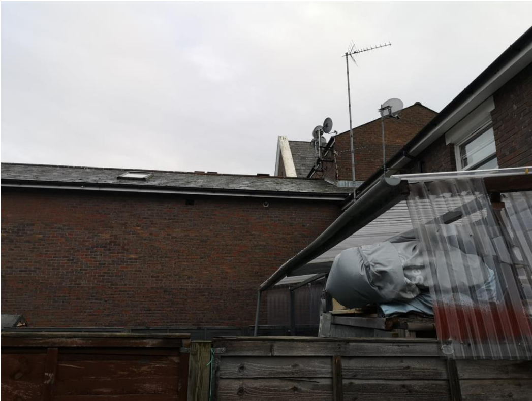
View the rear elevation of no.25 Lockesfield place
